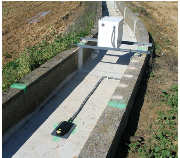
SonTek/YSI Argonaut-SW deployed in an irrigation canal.
