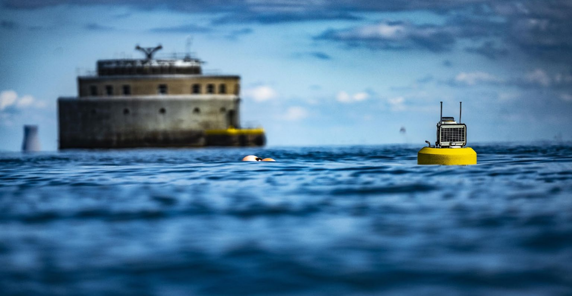
Toledo Water Intake Buoy
