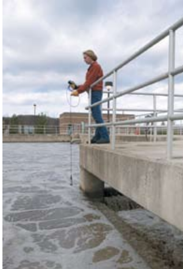
A typical wastewater sampling application in the aeration basin.
