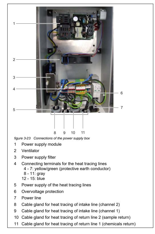
11 Unscrew the nuts of the cable glands for the cables of the heat tracing at the underside of the power supply box.
