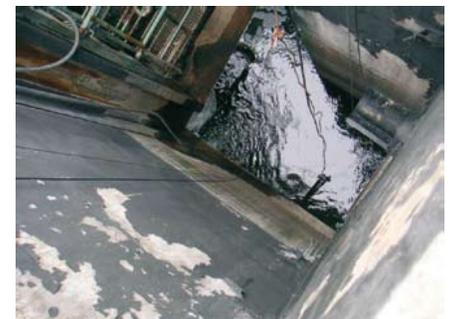
The ultrasonic cleaning capabilities of the ViSolid® and VisoTurb® prevents fouling of the optical sensors. They are installed here in a clearwell to monitor the plants effluent.
