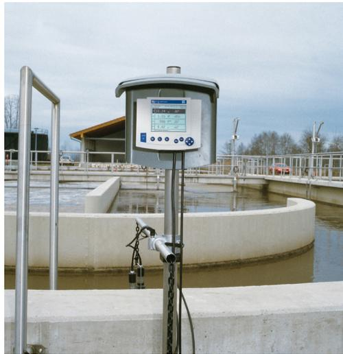
The IQ SensorNet 2020 XT terminal mounted tank side provides continuous process monitoring and control.
