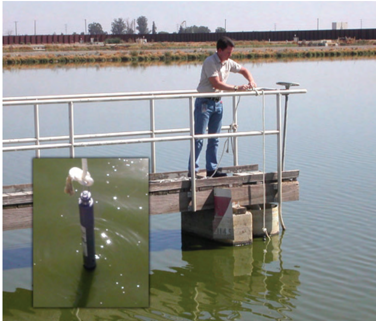
Deployment of a YSI 600 OMS Sonde with ROX DO sensor in a settling pond at the Sacramento, CA WWTP.
