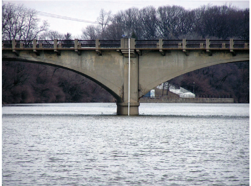
Deployment site for Indianapolis OES. The sonde is deployed in a long PVC tube for protection. The solar panel and telemetry system can be seen at bridge level.
